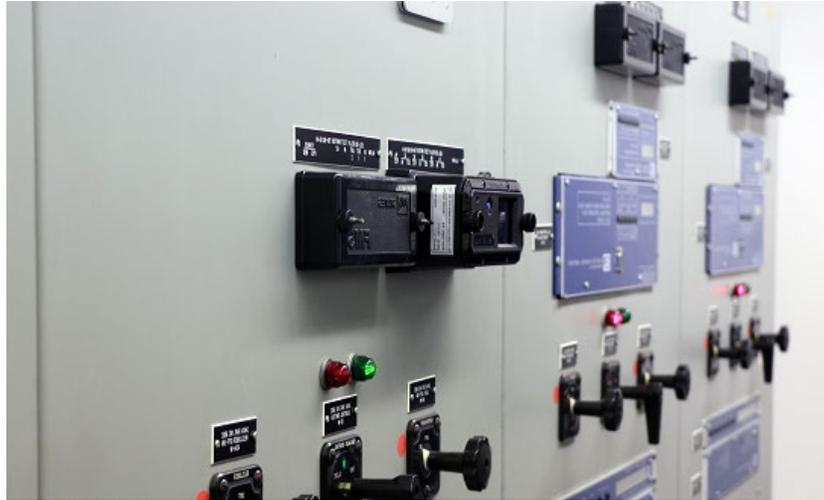
*38 SMART Block® devices worked together to simultaneously capture 45 waveforms on 5 buses and 40 circuits during a fault event. (Source: Fischer Block, Inc).*
